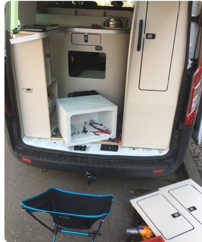
work in progress
